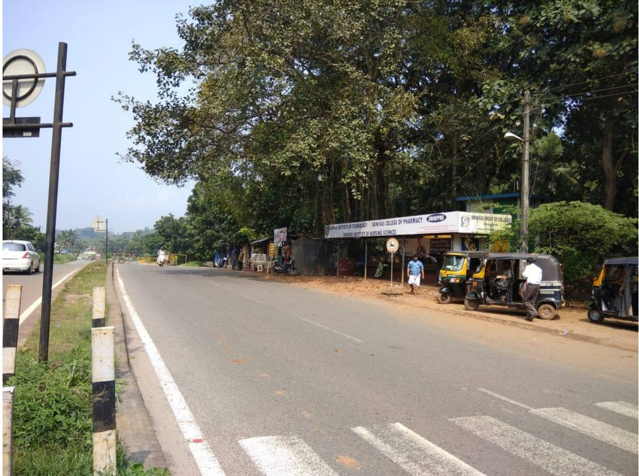
Bus Waiting Shelter on left side of Mangaluru-Bengaluru National Highway NH 75
