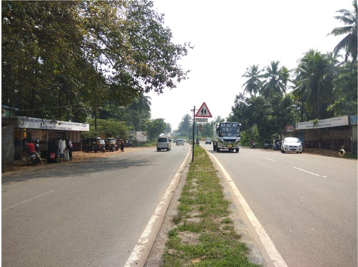
View of Bus Waiting Shelters at Valachil
