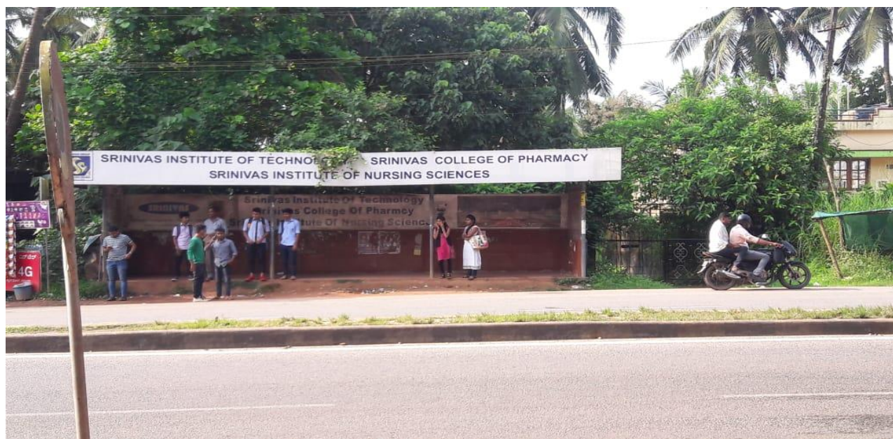
Bus Waiting Shelter on right side of Mangaluru-Bengaluru National Highway NH 75
